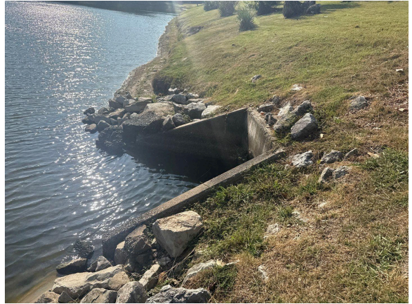
Lake concrete culvert
