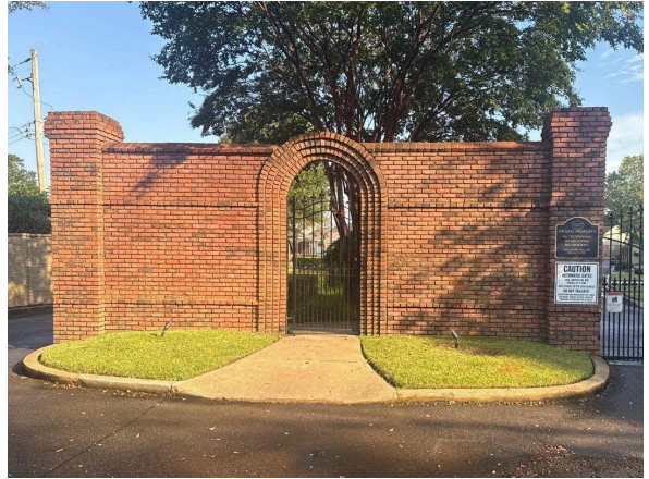
Entrance wall and gate
